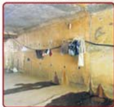
This cohort - now an abandoned bush dwelling - is one bathing area the peddlers use on the way to work.
